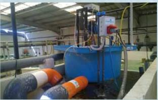
**Skim Plus** is a filtration control system by automatic foam adjustment.
